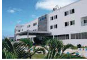
Rudrapur Plant (Green Building)
