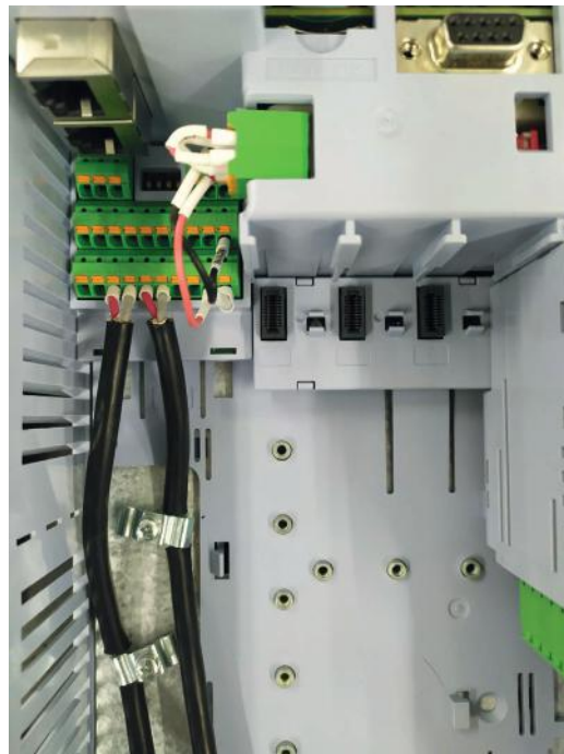
Figure 3.23: Connection example of control cable shield
