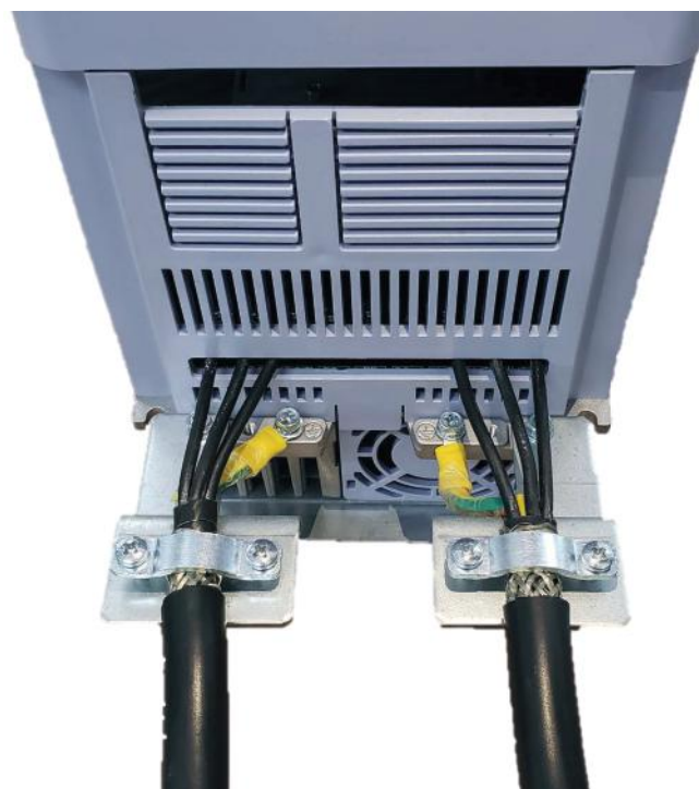
Figure 3.16: Detail of the motor cable shield connection
