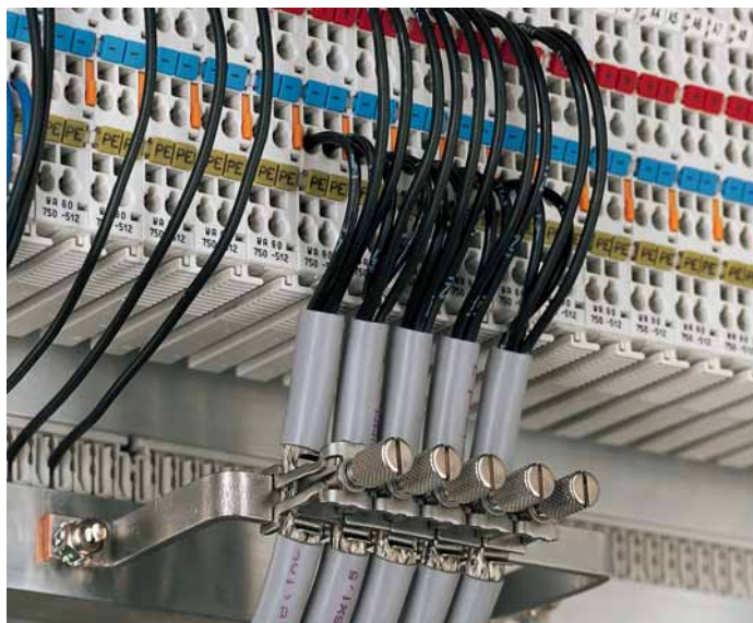
Figure 20: Application of the WAGO shield connecting system
